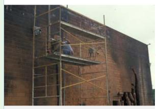
Even though an intense fire damaged this brick wall, the fire was categorically contained and the walls are worthy of testing for structural integrity and future use.
